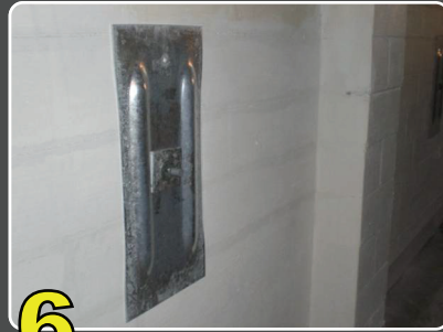
Wall Plate Attached
