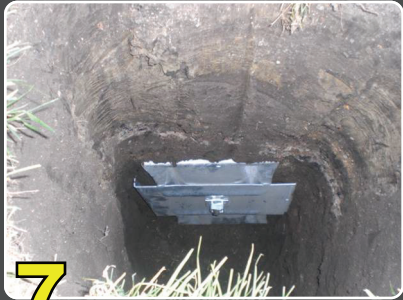
Anchor Torqued & Seated
