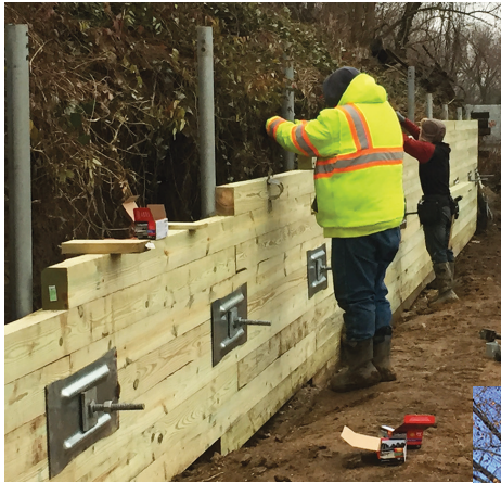
Continuing Placement of 4x6's
