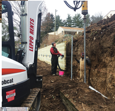
Installation of 34 Vertical Helical Piers and Setting the Wall.
