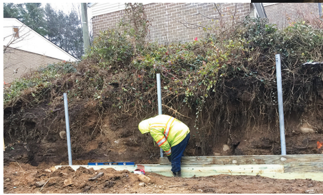
Setting the 240' Long Wall.
