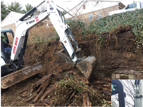
Demolition of Existing Failing Railroad-tie Wall.
