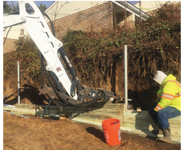
Installing Tiebacks
