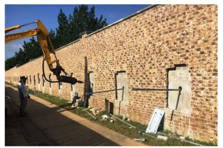
Residents of this high end neighborhood noticed cracks in the masonry retaining wall, but it was four years before repairs were scheduled. A lawsuit was filed against the developer because clay soils on the filled side were specified to be removed and replaced with soil. non-expansive geotechnical investigation of confirmed the site that expansive clay soil still existed behind the wall.
