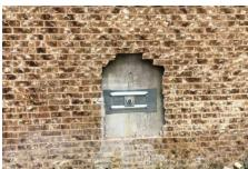
The project was very successful. As pressure was gradually applied to the wall over a three day period the wall rotation was corrected ranging from 3/4 inch to one inch. The repair has been monitored for a year and with no measured movement.
